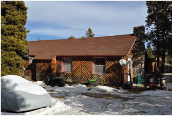
Figure 3.6. This cabin at 33436 Coal Creek Canyon Drive (5BL.11016) is atypical of most of Wondervu's Rustic-style cabins because it has decorative split-log siding as well as a stone hearth and chimney. (Photograph by Adam Thomas.)
