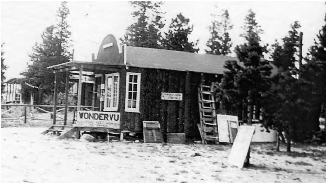
Figure 3.4. This building was probably the Wondervu land office as depicted on the Wondervu Project plat map (Map 3.2). The image probably dates to the 1930s. (Adeline Ortiz, Wondervu Café .)
