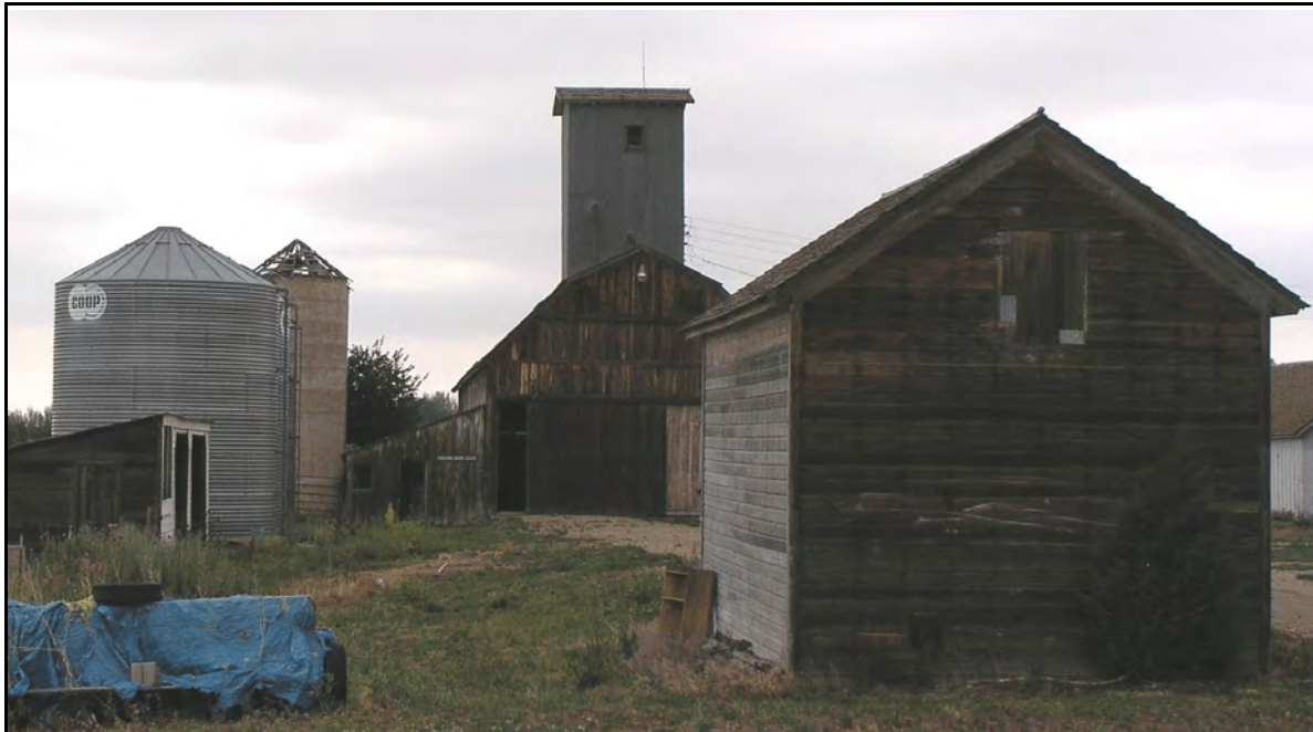
An evolution of grain storage structures can be found at 7016 N. 73 rd Street, including a granary, concrete stave silos, and prefabricated metal bins.
