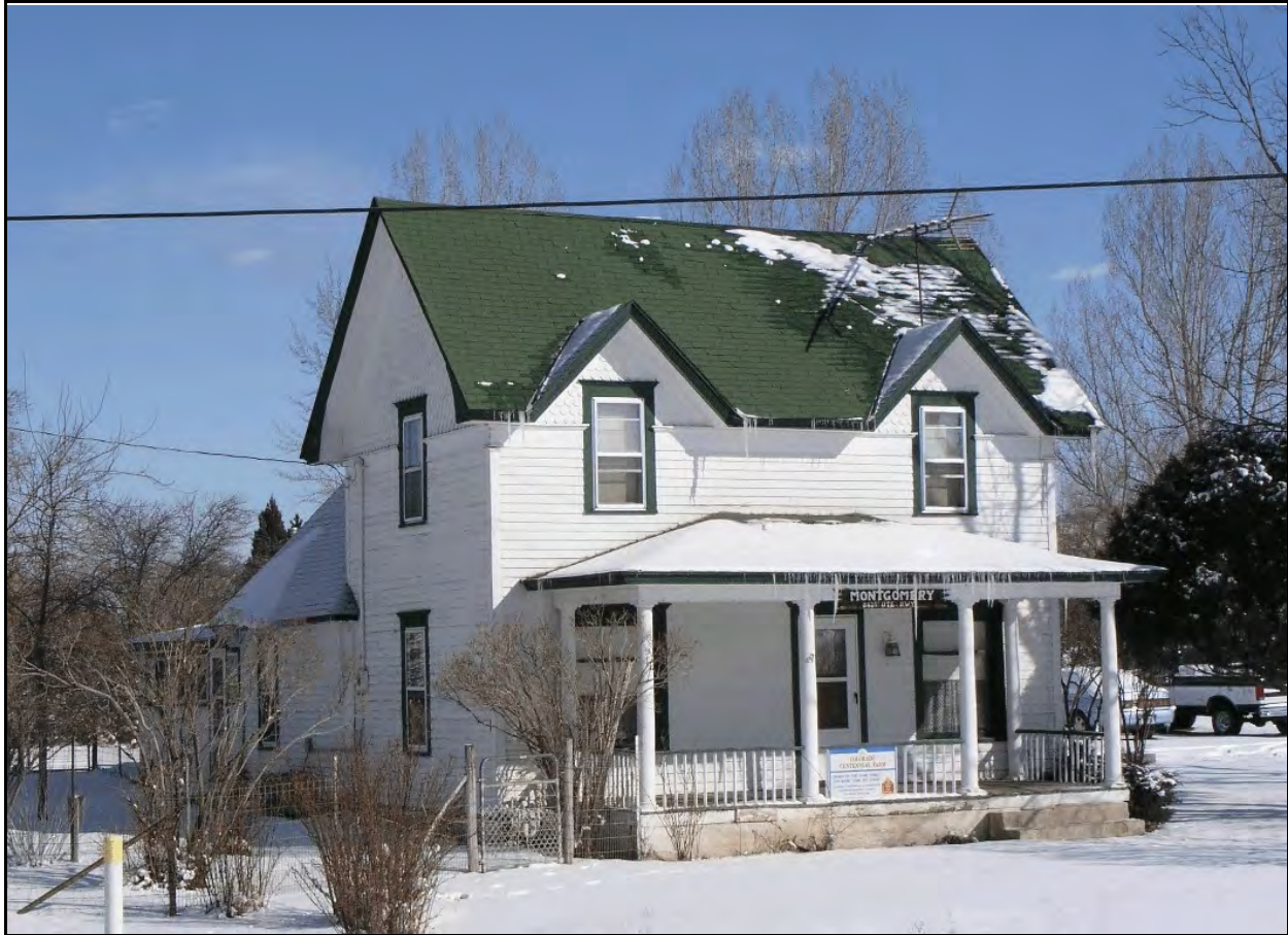
Farm house at the Montgomery Farm at 5486 Ute Road, a Colorado Centennial Farm. A basic I-house form, with additions and architectural detailing from both the Late Victorian and Early Twentieth Century revival periods.
