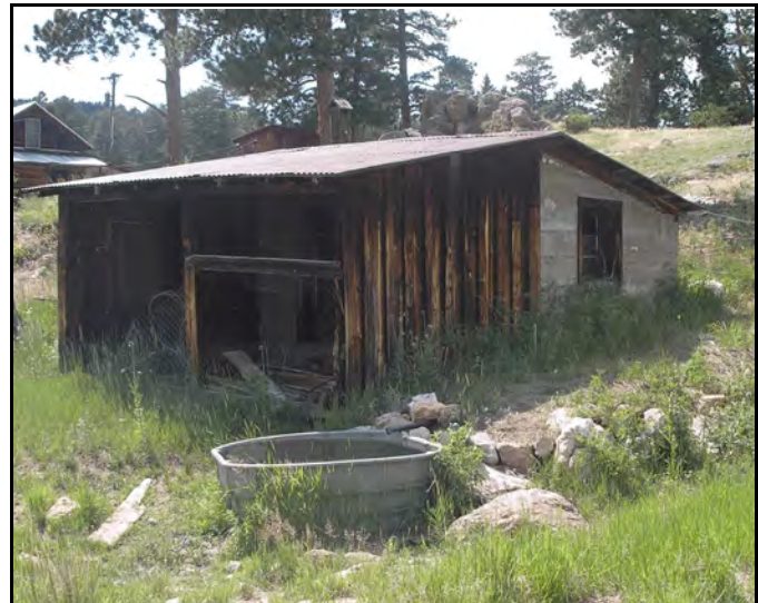
Concrete block springhouse built into the hillside at Scates Ranch, with a pipe leading to a stock tank.
