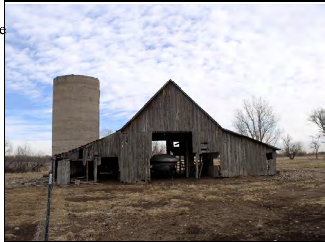
The Henning Farm barn – a Midwest three-portal barn formed by shed additions to the side. Photo by Carol Beam, BCPOS.
