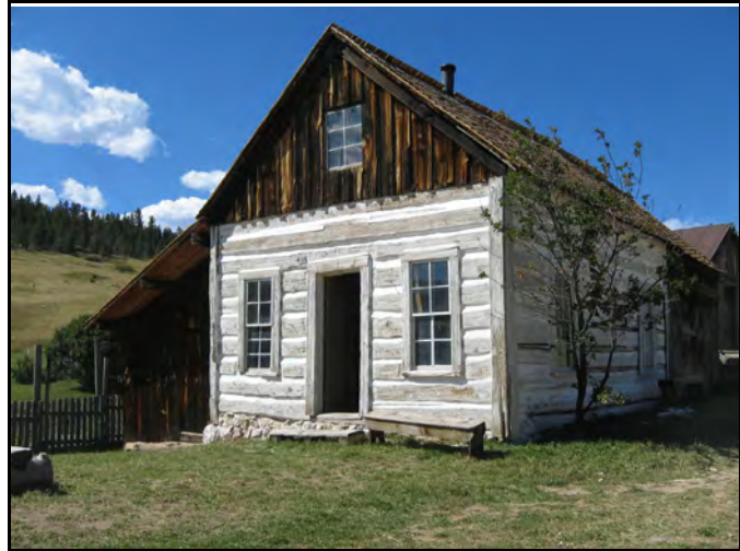
Walker Ranch log house, with squared log construction. Photo by Carol Beam, Boulder County Parks & Open Space Department (BCPOS).
