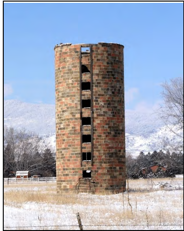
Hollow glazed clay tile silo
